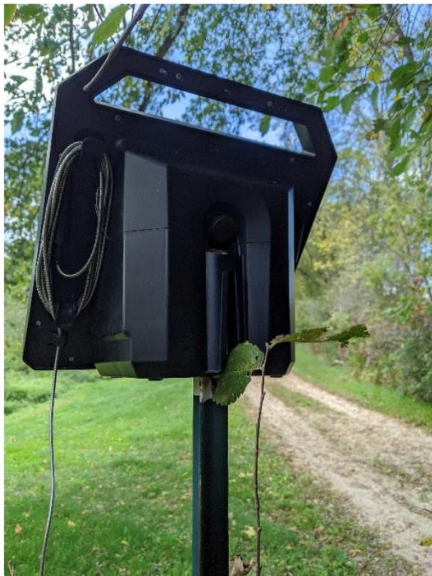
Rotate the unit so that it is facing the direction where it will get the most hours of sunlight during the day. Then lower it onto the post until the post is fully inserted in the slot. Gravity will hold the unit on to the post.
